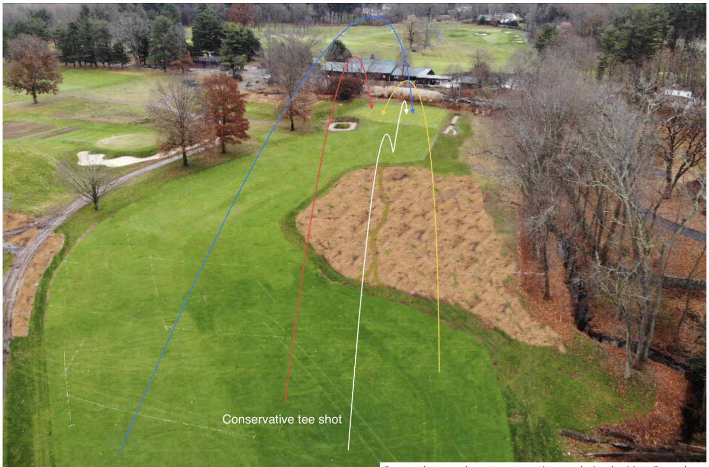
Drone photo and post-construction rendering by Matt Dusenberry
