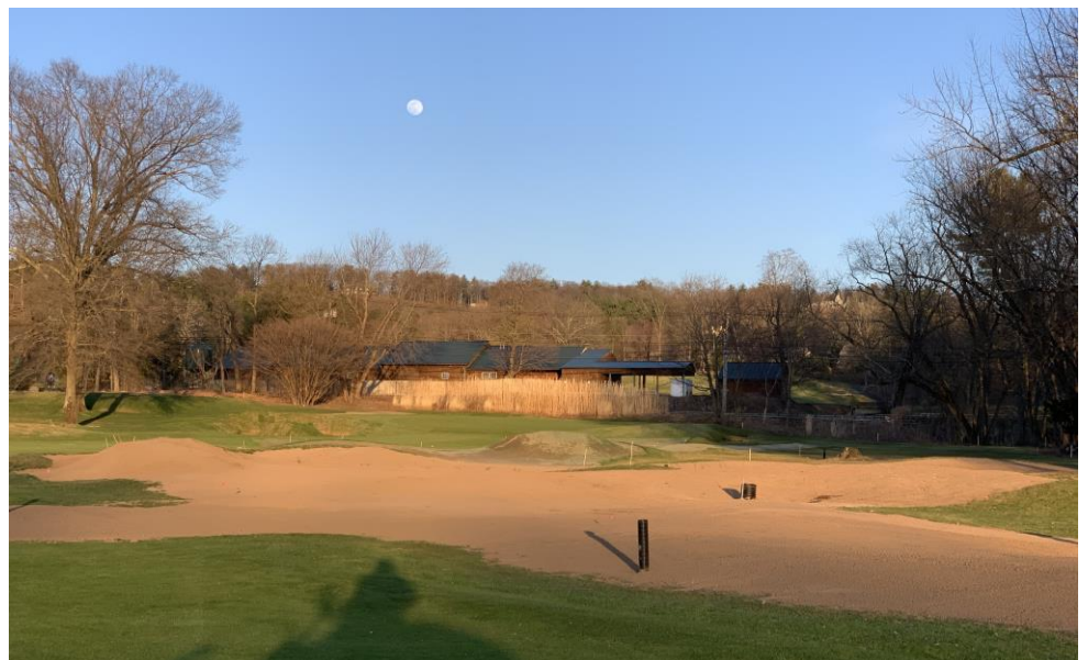
Renovated 13th hole, ready for hydroseed. Expanded fairway in the foreground. Hillocks and mounds just beyond. (photo - S. Ramsay)
